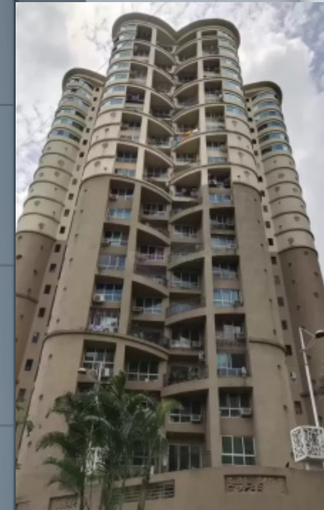
NAHAR OFFICE BUILDING (CHANDIVALI)
