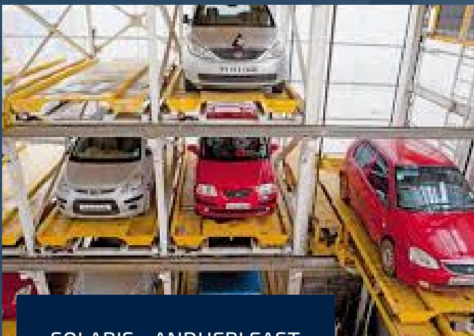
SOLARIS - ANDHERI EAST ROBOTIC PARKING
