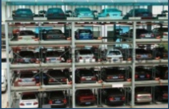
PUZZLE PARKING OF -3 AND 8 LEVEL ABOVE GROUND
