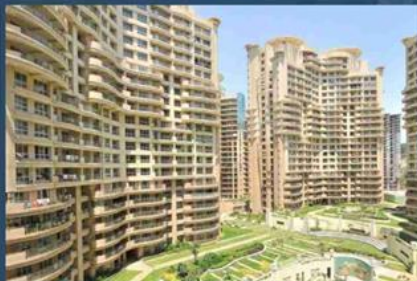
NAHAR 8 TOWER CHANDIVALI - ANDHERI EAST
