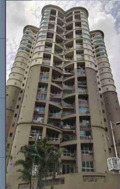
NAHAR OFFICE BUILDING (CHANDIVALI)
