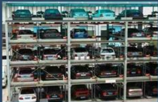
PUZZLE PARKING OF -3 AND 8 LEVEL ABOVE GROUND
