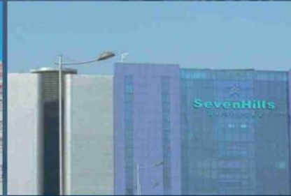
SEVEN HILLS HOSPITAL ANDHERI EAST, MUMBAI
