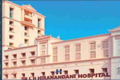
HIRANANDANI HOSPITAL POWAI, MUMBAI
